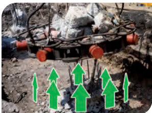
Lifting up, PB takes out the concrete and leaves the steel rods free
