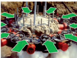
Activating the oilflow, PB crushes the concrete part without damaging the lower structure
